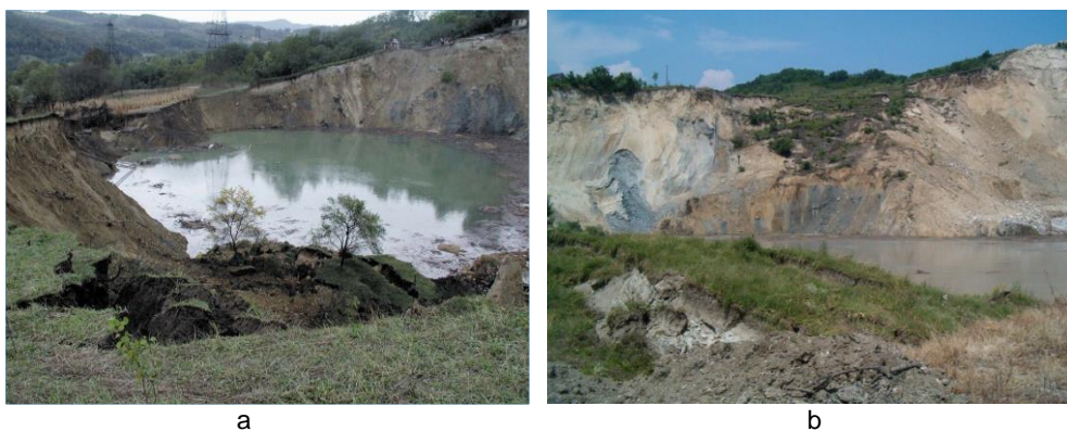
Fig. 3 The implosion of the brine caves at Ocnele Mari: a - the cave from 2001; b - the cave from 2004 (Luca and Tigaret 2008).
