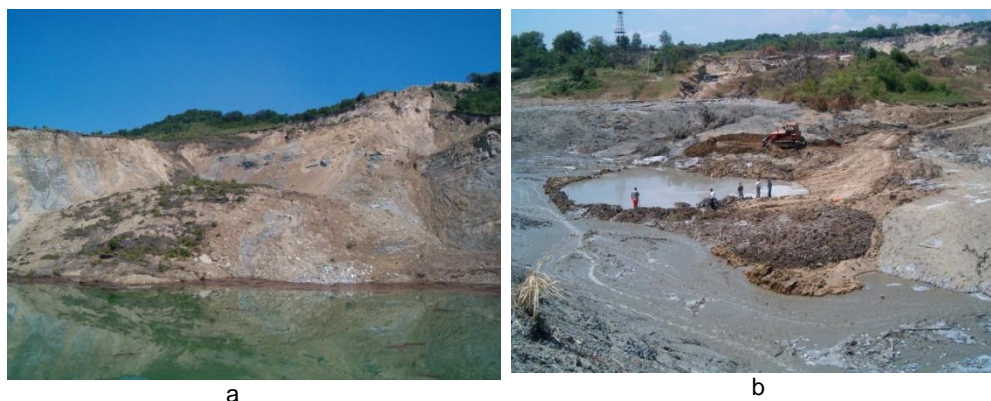
Fig. 7 The condition of the slope affected by the implosion of the caves in 2005: a - implosion cone and subsidence with brine lake (photo Luca, 2008); b - the development of caves by the collapse of the banks.
